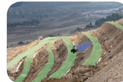
Visual inspection of installations
